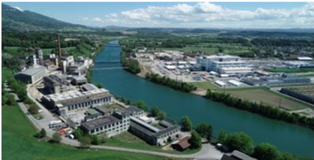
Figure 1: Ex-wood-processing factory area in Riedholz/Luterbach, Canton of Solothurn (2012).
